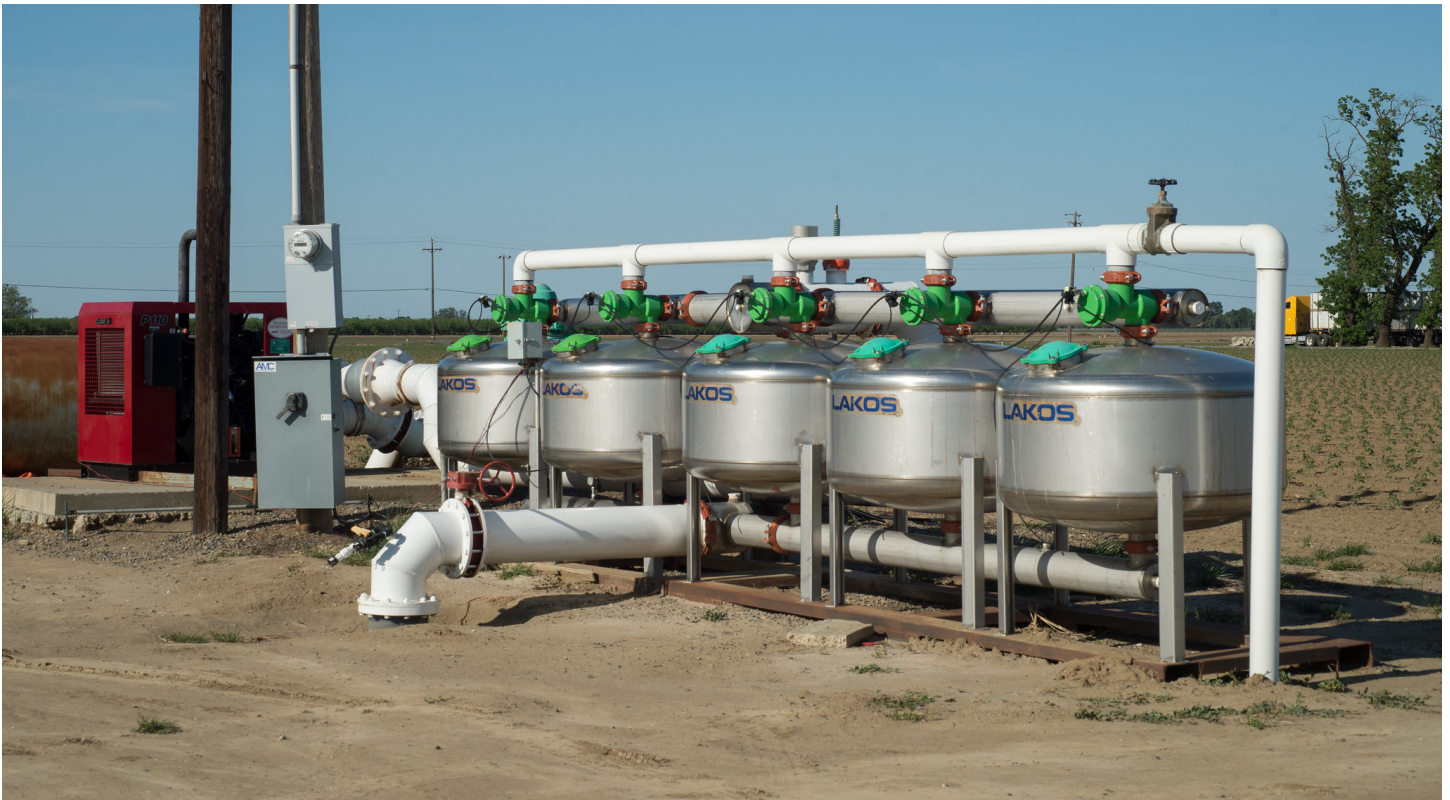
EQIP-funded water filtration and drip irrigation system on California tomato farm, USDA .
