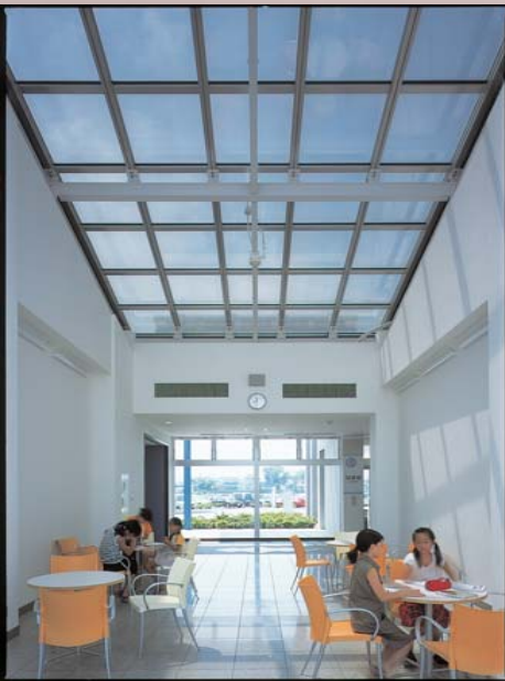
Cultural Center, Gyoda City, Saitama Prefecture, PV Atrium Glass
