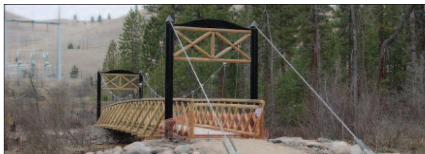
Small-diameter-wood bridge near Missoula, MT.
