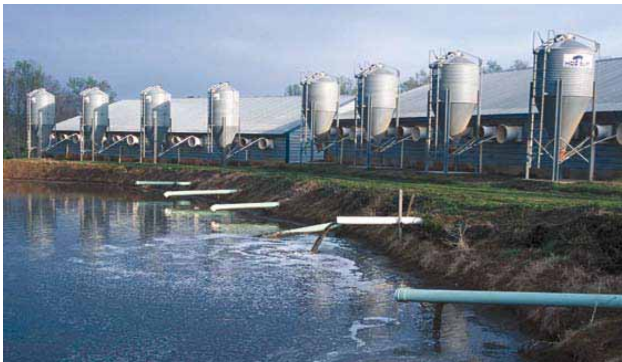
State of the art lagoon waste management system for a 900 head hog farm. The facility is completely automated and temperature controlled – United States 2002
