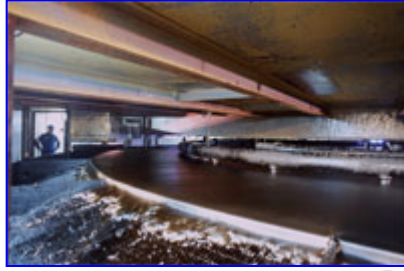
Tar Sands Extraction Separation Cell, Alberta, Canada
