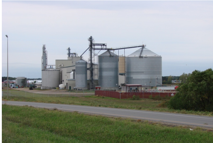
Central MN Ethanol Plant
