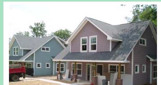
The Blacksburg duplex project utilizes pervious paving systems and other sustainable site features.
