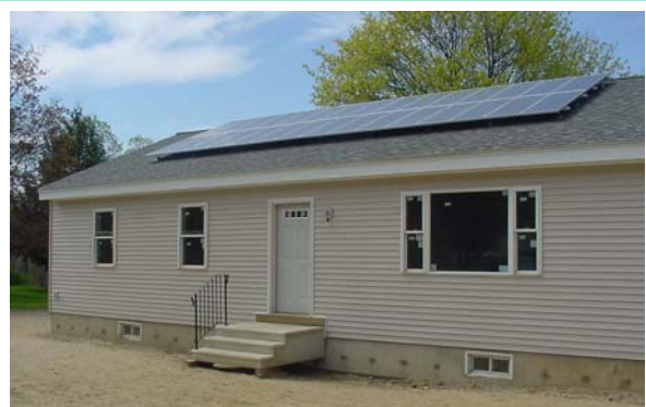
RDI submitted this single-family house for green certification under the LEED-H rating system.
